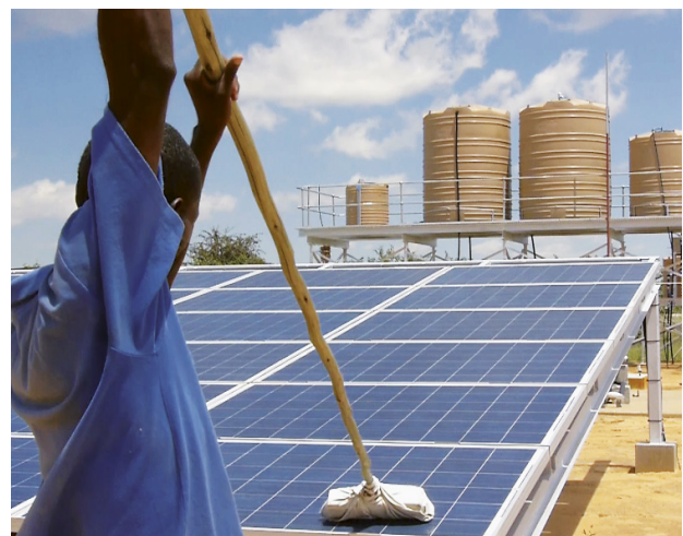
Desalination plant: Cleaning the solar panels
