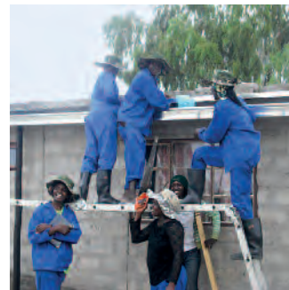
Local trainees preparing a roof for rainwater harvesting
