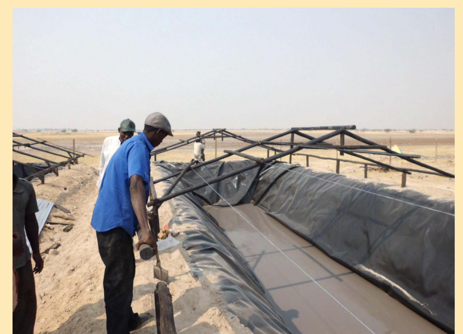
Figure 4: Training of local users in the construction of water storage tanks
