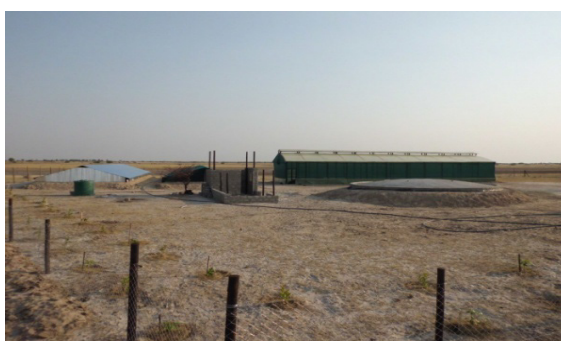
Fig. 4. Option 3: Flood water harvesting with storage of surface water from Oshanas in a combination of underground tanks and ponds (Iipopo)
