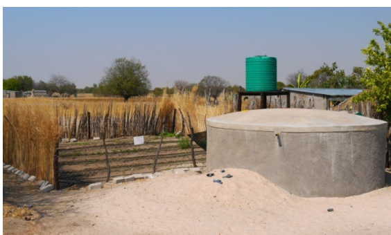
Fig. 2. Option 1: Rainwater harvesting with ferrocement tank (Epyeshona)
