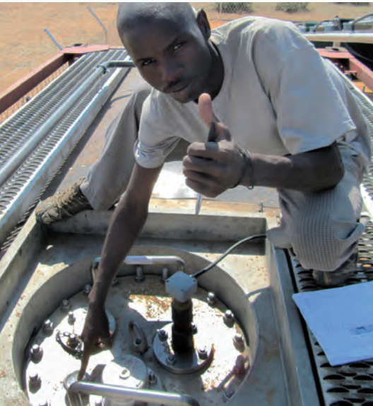
Festus checking the desalination plant
