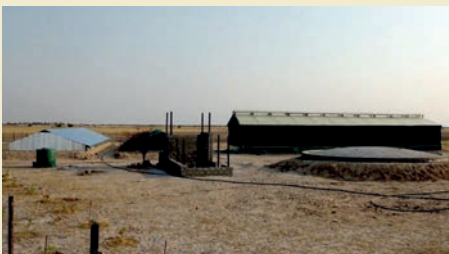
The pilot plant for subsurface water storage in Iipopo
