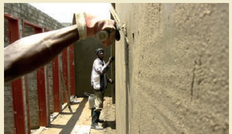
Construction of communal washing house
