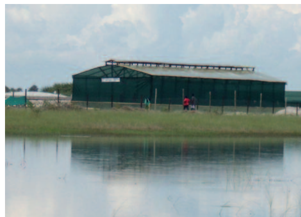
Floodwater harvesting pilot plant at Iipopo next to an Oshana
