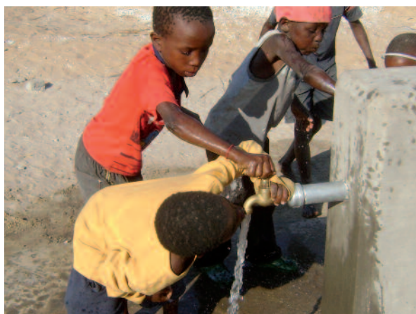
Children at the groundwater desalination plant
